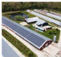
Commercial and Industrial Solar Projects
